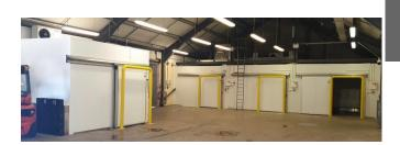
The initial part of the job was to dismantle the existing cold rooms, decommission the refrigeration systems and remove them from the site. The new cold rooms were installed and then all the new refrigeration equipment and the control panels. The final part of the contract was to relocate an ice-flaking machine to operate above the new freezer room which would allow the flaked ice to drop via a chute to storage bins within the freezer room.
